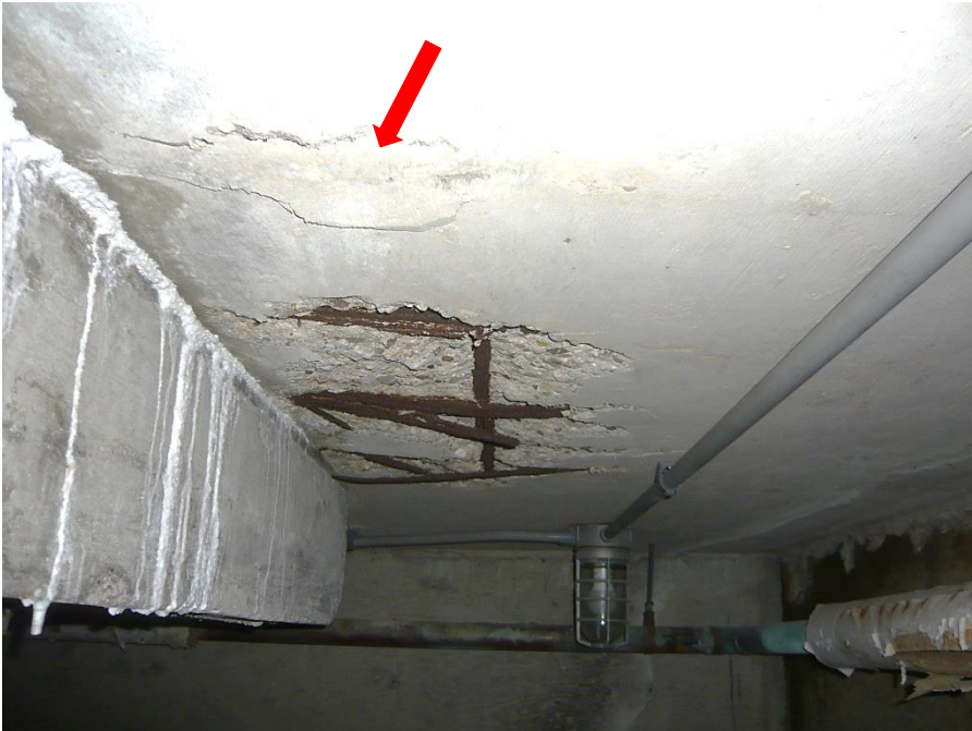
Figure 8: Typical view of an open spall on the underside of the pool deck slab with exposed corroded steel reinforcement. Arrow indicates an incipient spall (loose overhead concrete) adjacent to the spall
