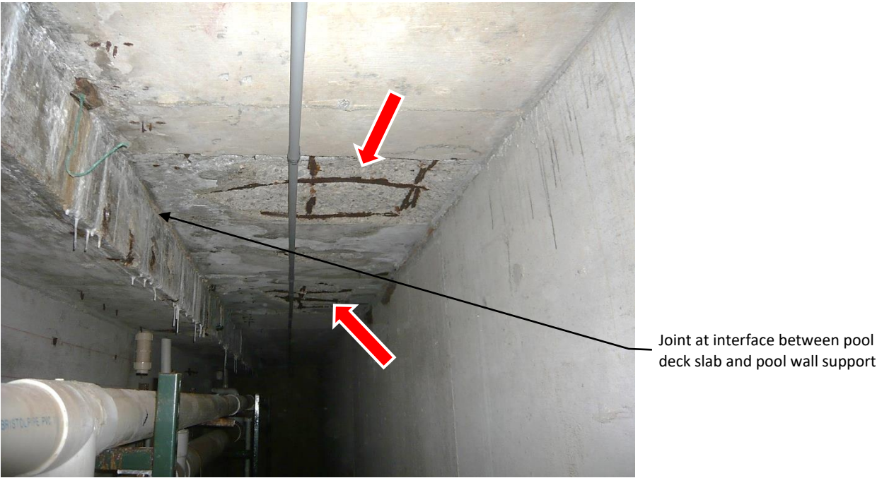
Figure 2: Spalled concrete, with exposed corroded steel reinforcement, on the underside of the structural pool deck slab. Note efflorescence staining (white mineral deposits), an indication of previous and/or active water infiltration, along the length of the slab to pool wall support interface.
