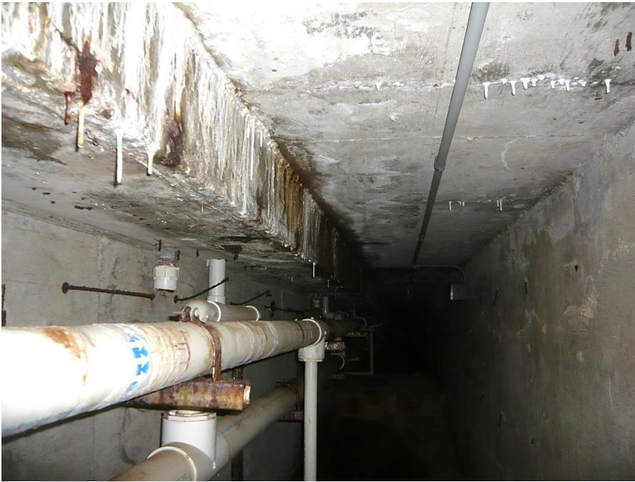
Figure 11: Typical view of efflorescence staining (white mineral deposits), an indication of previous and/or active water infiltration, along the length of the slab to pool wall support interface.
