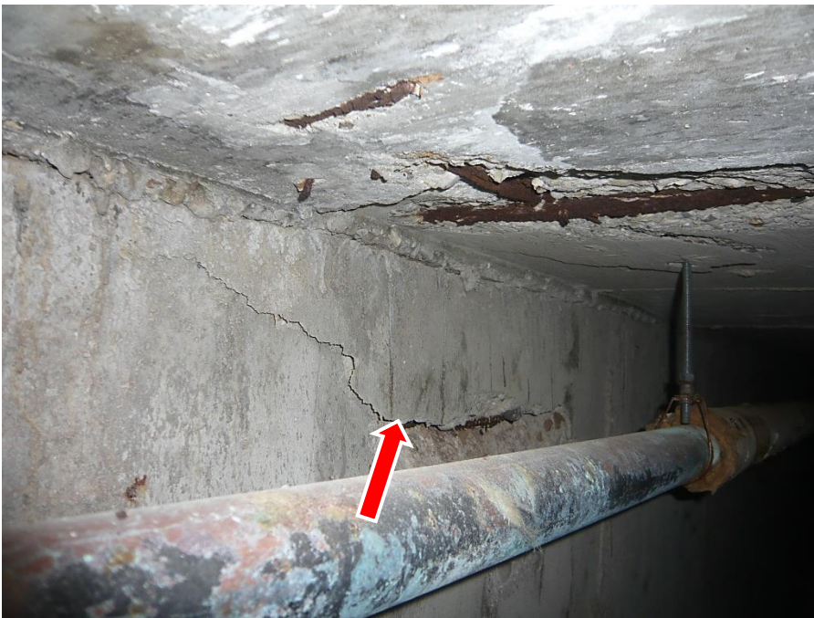
Figure 6: Incipient spall (loose overhead concrete) at the building foundation wall as observed near the center of the north edge of the pool. Note, spalled concrete with exposed steel reinforcement on the underside of the pool deck slab
