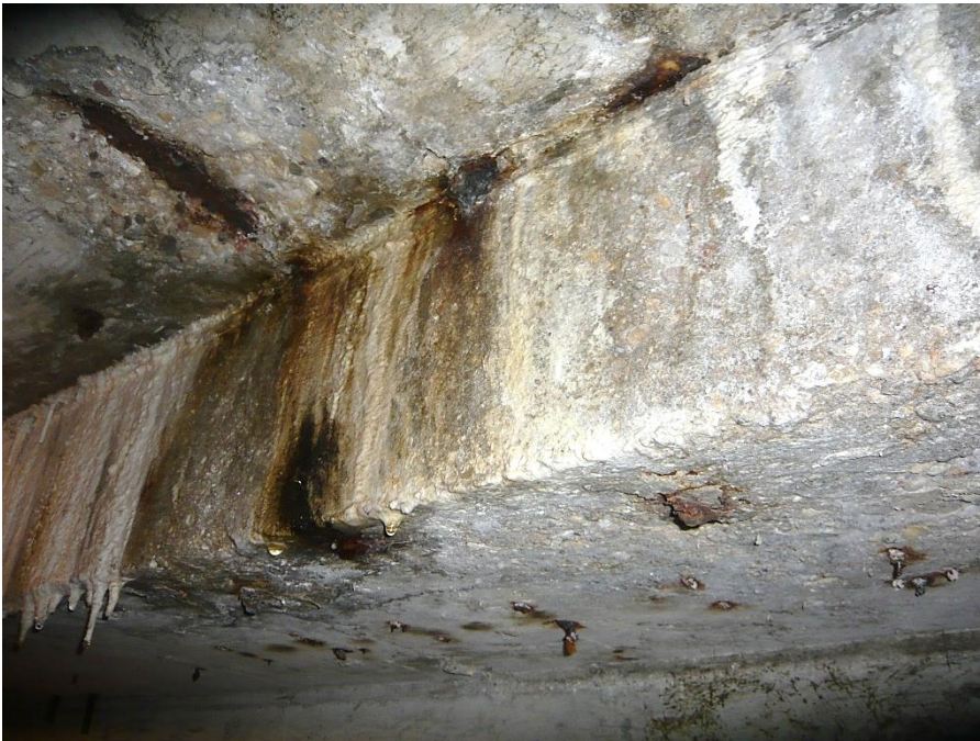
Figure 10: View of active water leak and efflorescence staining at the slab to pool wall support interface.
