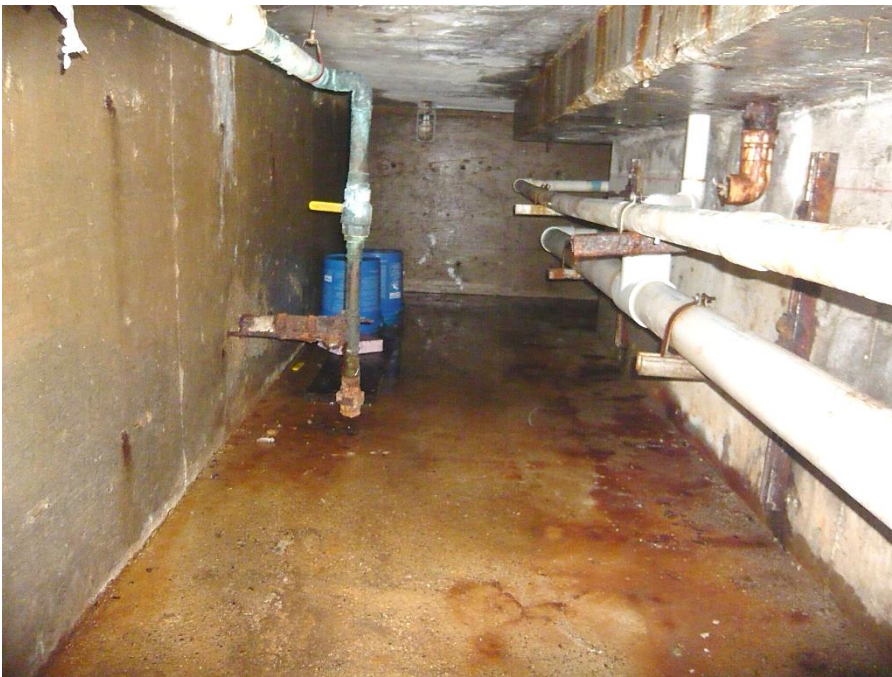
Figure 12: Standing water on the tunnel floor slab at an area of an active water leak as observed at the southwest corner of the pool
