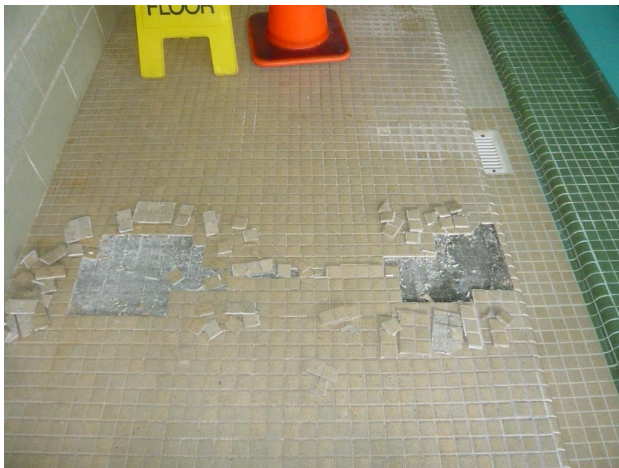
Figure 15: Debonded tile near the southwest corner of the pool. No unsound concrete was visually observed or detected via hammer sounding where exposed
