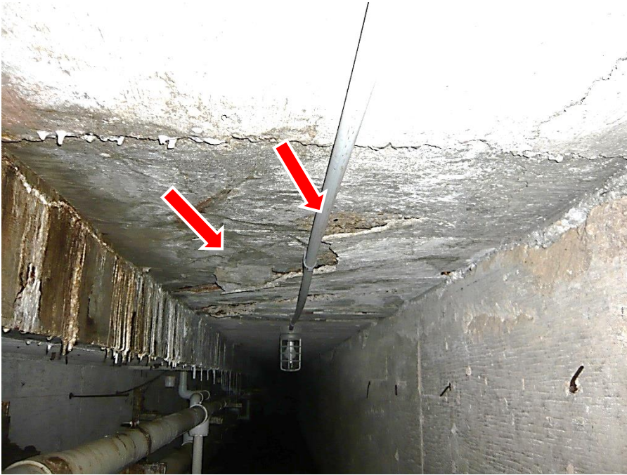
Figure 7: Incipient spall (loose overhead concrete) on the underside of the pool deck slab as observed along the south edge of the pool
