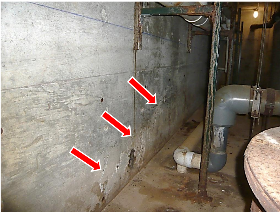
Figure 4: Incipient spall (loose concrete) at the base of the pool wall as observed along the north edge, near the west corner of the pool
