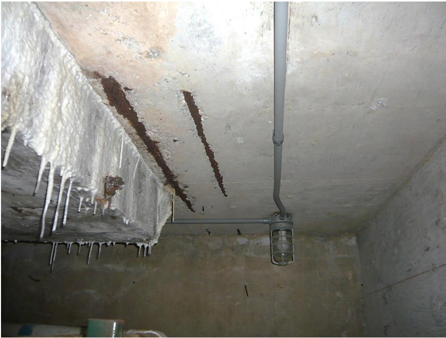
Figure 9: View of corroded steel reinforcement placed at the bottom surface of the pool deck slab. Sounding of adjacent areas did not indicate areas of unsound concrete
