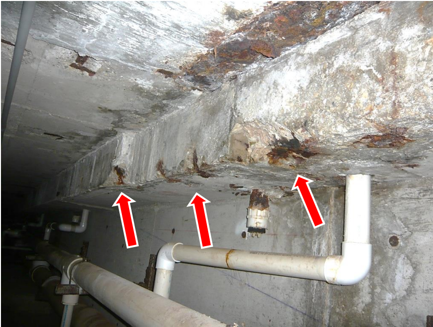
Figure 3: Spalled concrete, with exposed corroded steel reinforcement, on the underside and face of the portion of the pool wall that supports the pool deck slab
