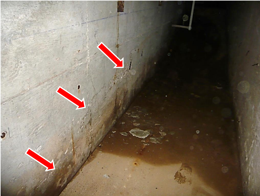
Figure 5: Incipient spall (loose concrete) at the base of the pool wall as observed near the center of the south edge of the pool
