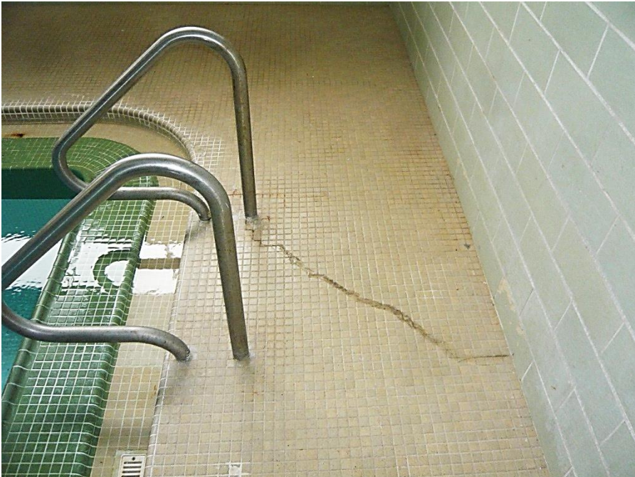
Figure 14: Cracked tile and grout joints, previously filled with a caulk material, as observed near the southwest corner of the pool
